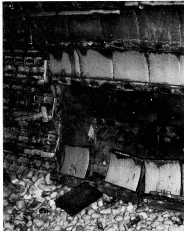
Fig. 10—'White iron' blocks during removal
